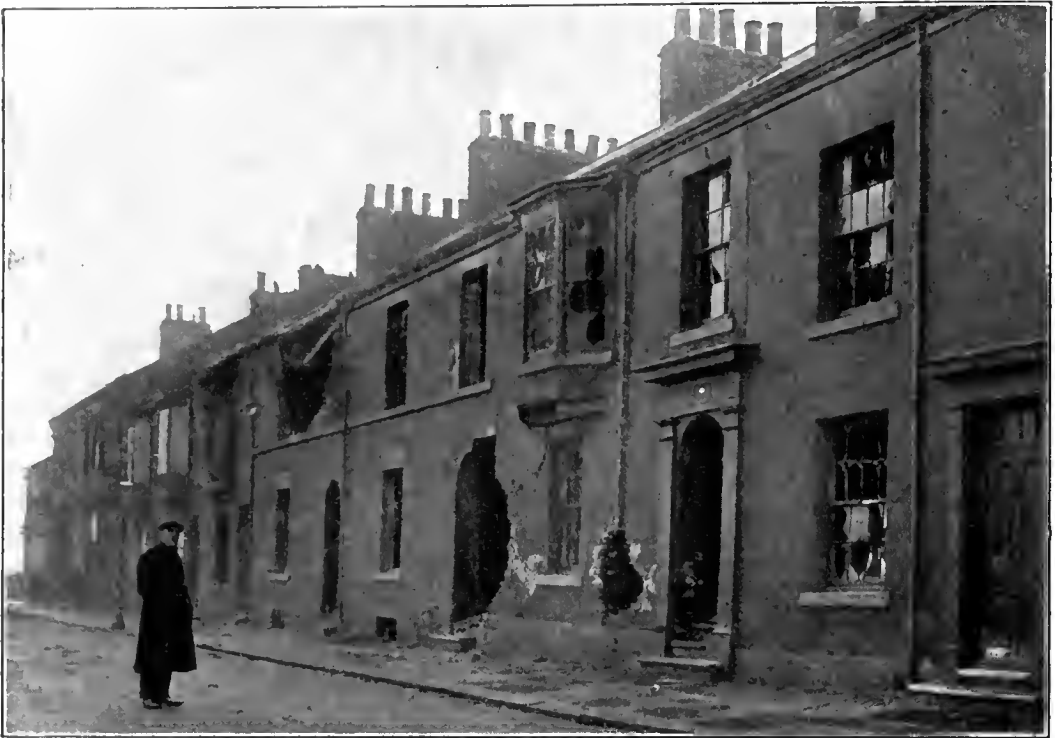
HARTLEPOOL: VICTORIA PLACE. Practically the whole of this street was wrecked.
